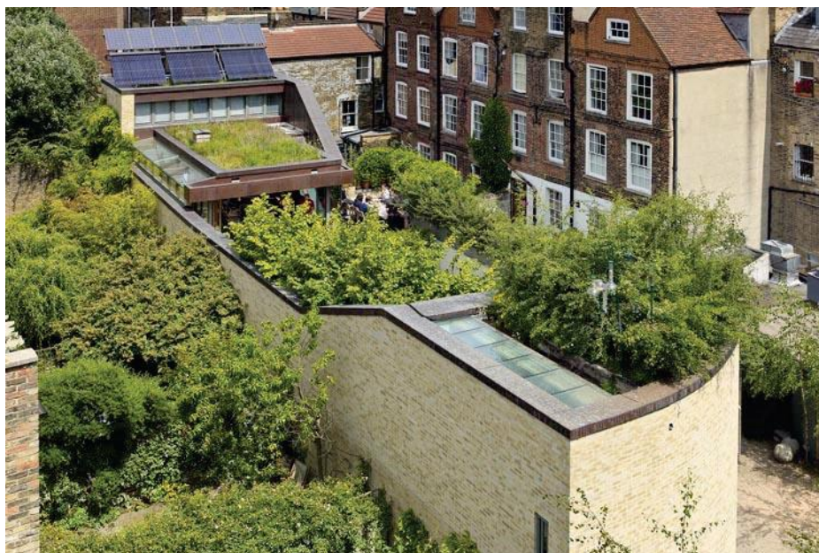
Figure 62 Terrace with Green roof
