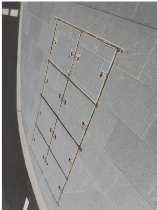
Figure 155 Typical service pit treatment
