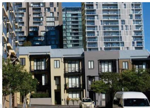
Figure 70 Terraces, Pyrmont Source: THSC
