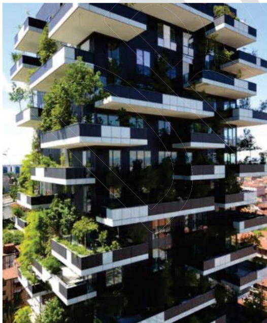
Figure 31 Greened Residential Flat Building, Bosco Verticale
