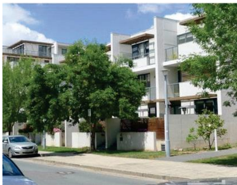
Figure 67 Terrace style housing, Kingston Source : THSC
