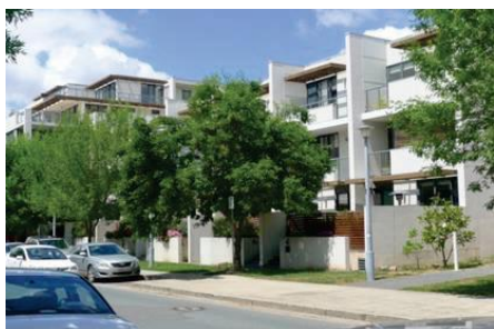
Figure 54: Elevated entries allow for surveillance and privacy
